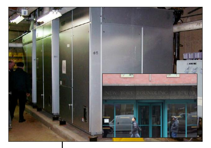
Since the chiller plant is made up of three modules it is easy to stage the load while offering more redundancy than a single chiller system. The Yazaki chiller produces low noise and no vibration. This lowers the installed cost as expensive machine room sound attenuation is eliminated and vibration isolation is not required. These features are critical performance factors for an acoustically sensitive project such as a hospital.
